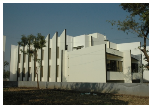
IAS / IPS Centre (Under Construction)
